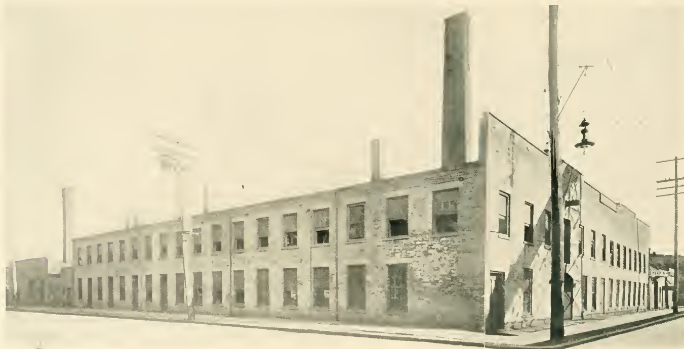
NEWARK CHAMOIS CO., NEW JERSEY RAILROAD AVENUE.
